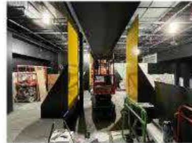
End cap panels installed.
